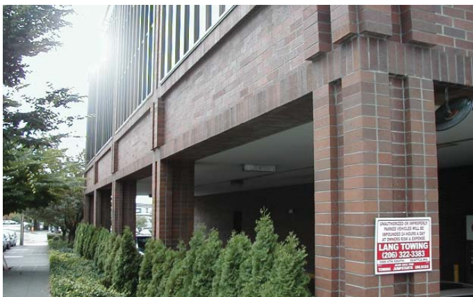
Figure 20 RHCM Columns and Spandrels Used Both as a Form and for Structure
