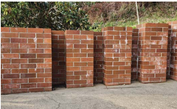
Figure 7 Articulated Retaining Wall
