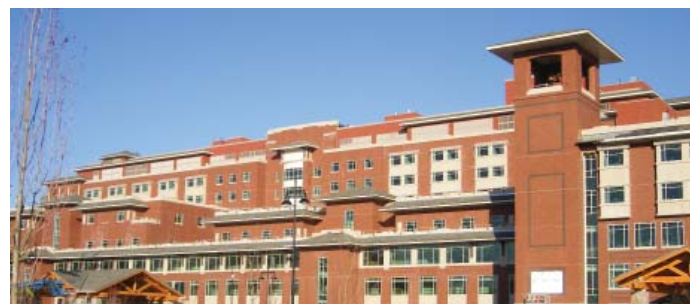
Figure 18 RHCM Reinforced Veneer Hospital Exterior Wall in a High Seismic Zone
