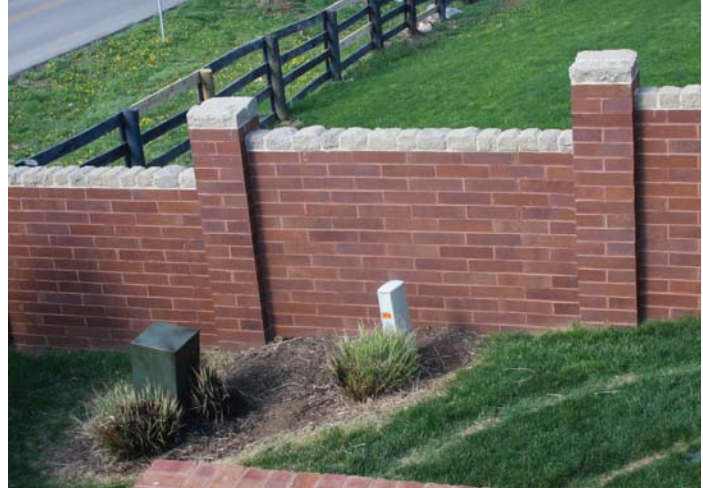
Figure 10 Pier and Panel Sound Wall
