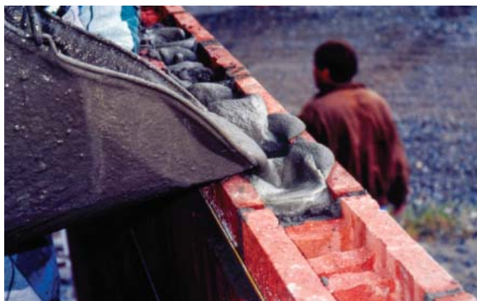
Figure 29 Fluid Grout
