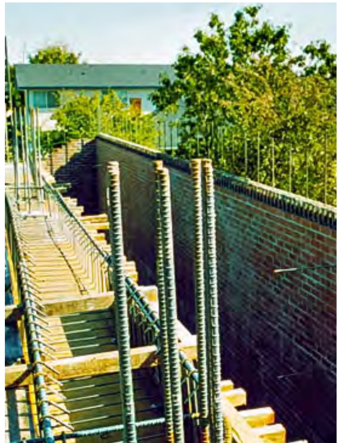
Figure 4 Reinforced Hollow Clay Masonry Wall with Shear Keys for the Slab Connection
