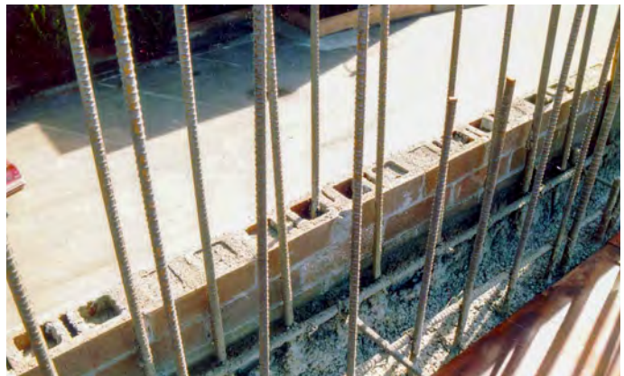
Figure 21 RHCM Used as the Finish Wall and Backing for Concrete Shotcrete (Gunite)
